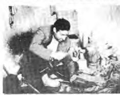
TO MAKE A STEEL FILE, Iranian bazaal style, you need a big toe to hold the metal a steady hand to make the ridges 1/3210 of an inch apart, and a charcoal fire and bucket of water for tempering purposes.
